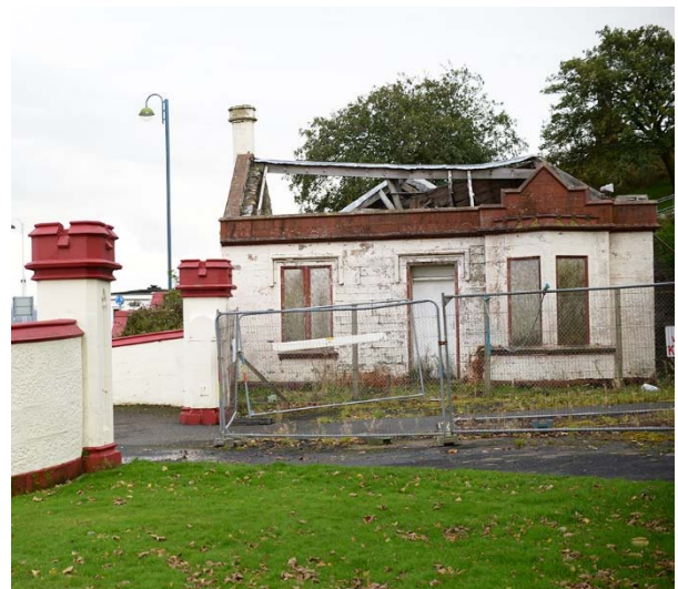
Castle House Gate Lodge
