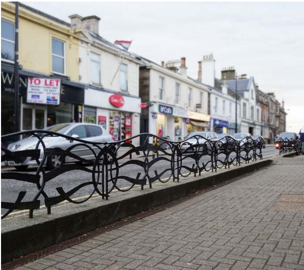
Barrier to pavement – Argyll Street
