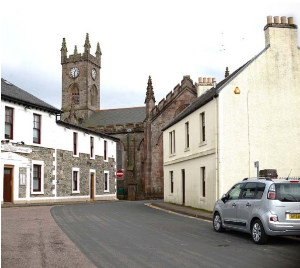
Kirk Street looking towards the High Kirk. The organic old street pattern reinforces the sense of old Dunoon (early 19 th Century) as a highland 'clachan' then a cluster of cottages arranged around the village church.
