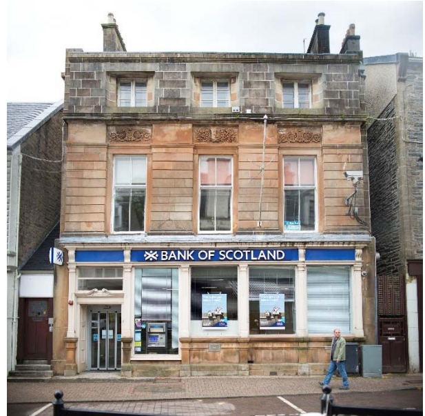
Photograph of the Bank of Scotland at 66 to 76 Argyll Street. A good example of where the original sash and case and casement windows play an important role in defining the character of the overall building.
