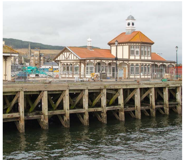
Waiting Room and Pier Masters Office from the quayside. Dunoon Pier - Clarke and Bell with Sir William Copland in collaboration with R A Brydon and C J M Mackintosh, 1896-98; incorporating earlier pier to N by Campbell Douglas, 1867-68 Largely retaining its original form and distinctive detailing, it is acknowledged as the finest Victorian pier building of its type in the country. It is of crucial importance to the Dunoon's historic character
